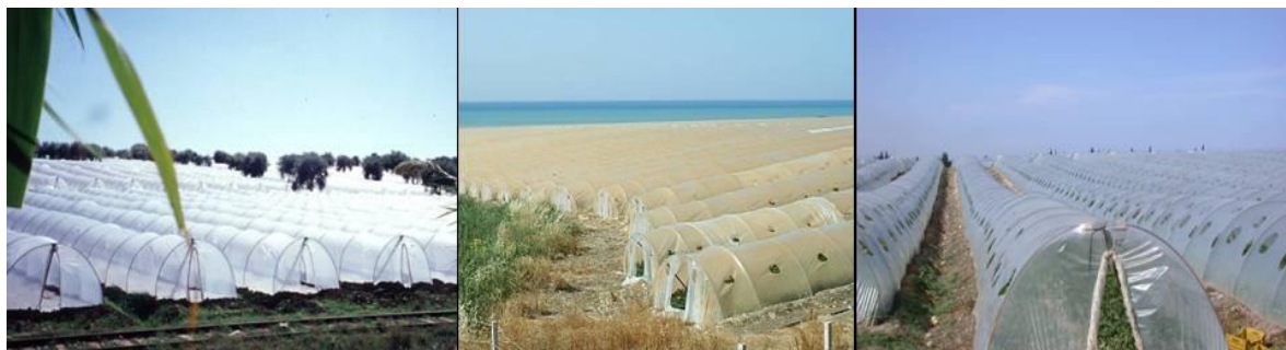
Figure 18: Seasonal manipulation of ventilation in tunnels in Sicily, IT. From left to right, winter, early spring, late spring. The next step is complete removal of the cover. Photos: Cecilia Stanghellini (left) and Giuseppe Noto (centre and right).
