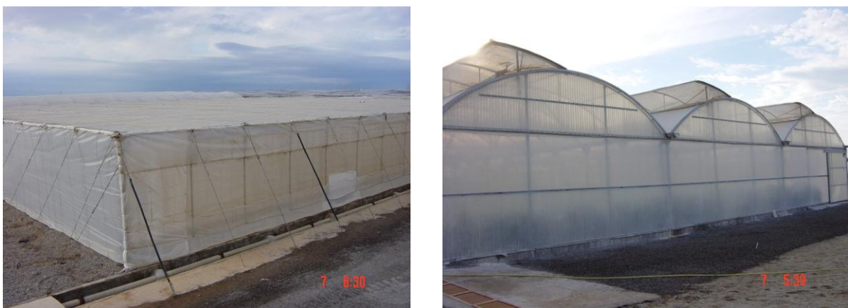
Figure 12: Examples of low-tech plastic greenhouse: the traditional low-cost ‘parral’ (left) and the more innovative pre-fabricated arch-shaped multi-tunnel (right) (photos: Alberto Pardossi).
